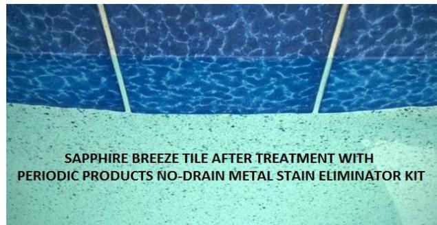
This particular tile has a small metallic content. The metallic content in the tile is reacting chemically when **Manganese** is present in the pool water causing the tile to turn black.
